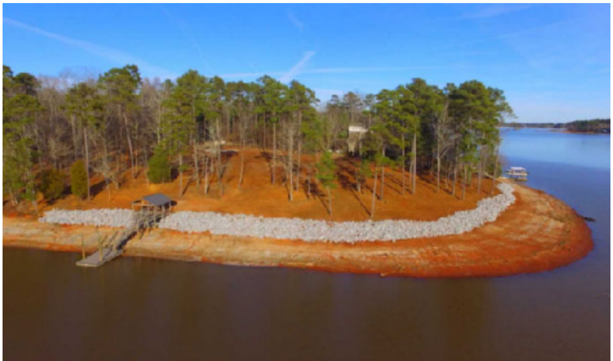
Shoreline adjacent to 288 Vinge Road after installing rip rap and brushing.
